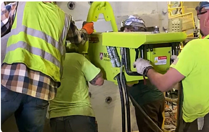
Installing the hammer with monorail positioning assistance.
