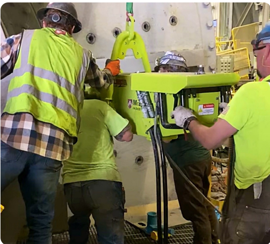
Reline crew installing the hammer.
